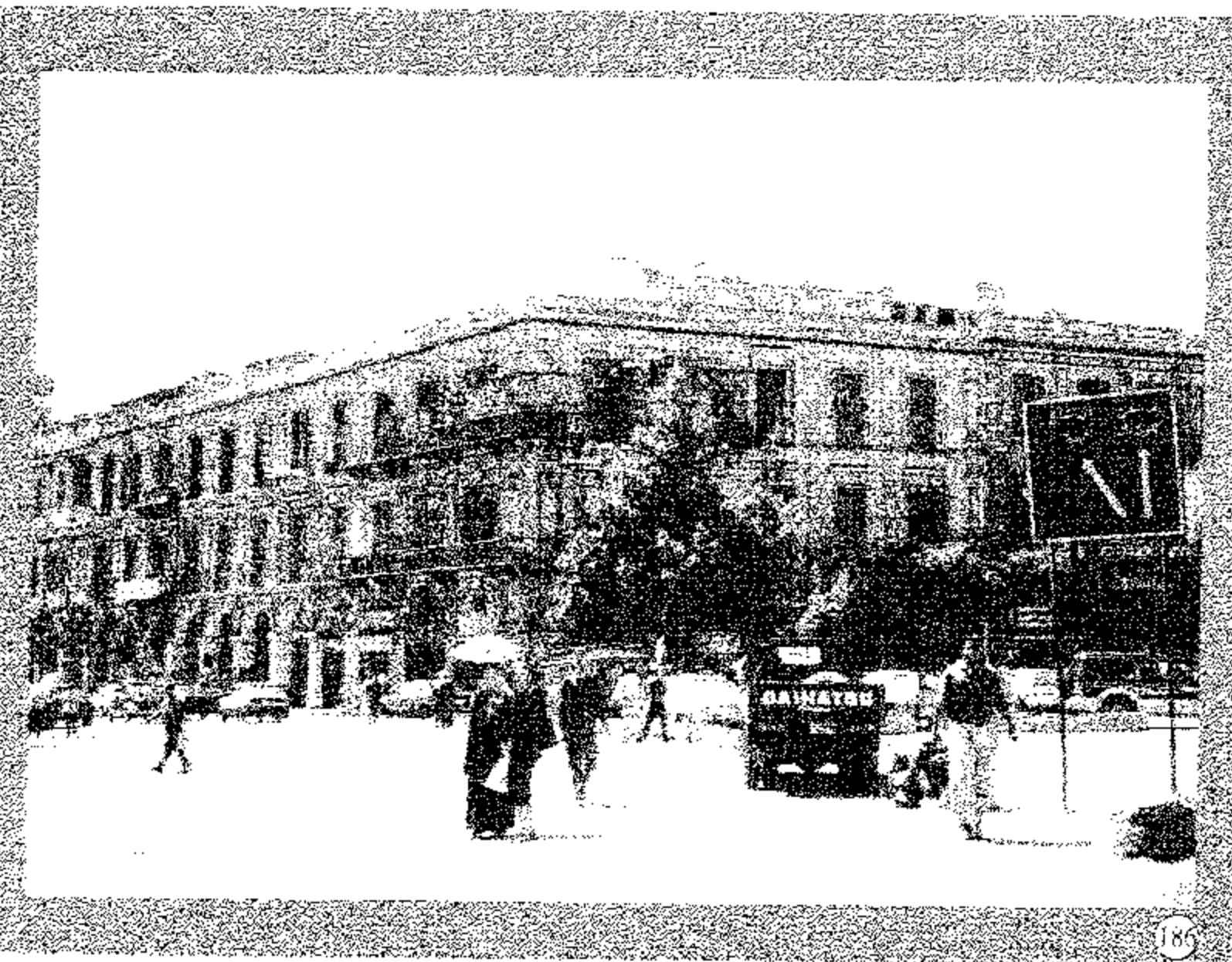
16 Aly El - Kassar St. (former El-Guneyna St.) Built : end of 19 th Century Area : 2250 m 2 No. of storeys : 3 (145 rooms) Style : Classic, among bldgs. with pedestrian arcades
